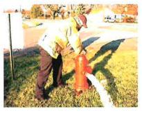
Additionally, Fire District personnel do periodic flow checks in new developments. One career Firefighter is assigned to tracking out-of-service hydrants. In 2005, nearly 30 hydrants were reported as damaged, leaking, or otherwise out-of-service; of those, only six remain out-of-service. Repairs needs are reported to the respective agency and are often addressed within days.
